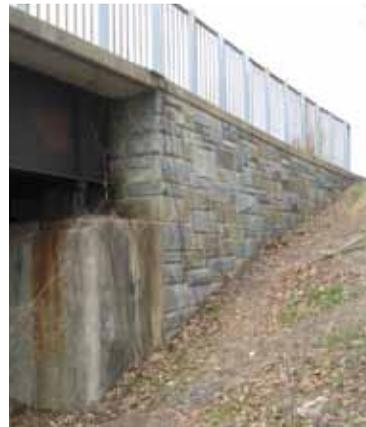
Stone cladding on bridge at George Washington Memorial Parkway (new guard rails in the Four Mile Run stream corridor should comply with guidelines addressing railings and handrails)
