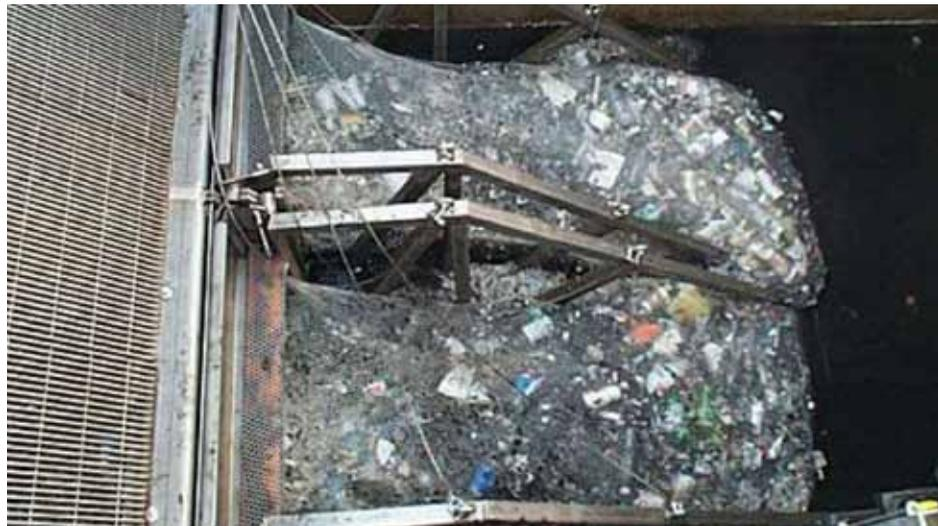
Example of a custom fabricated litter interceptor, detail/section above, photo below
