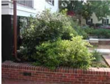
Stormwater planter connected to roof downspout
