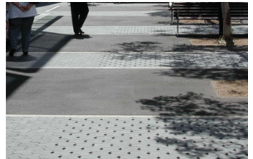
Examples of paving materials used in combination. Above, cast-in-place concrete, stone and recycled rubber; below, asphalt and permeable pavers
