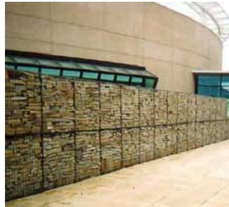
Stone and gabion clad concrete wall
