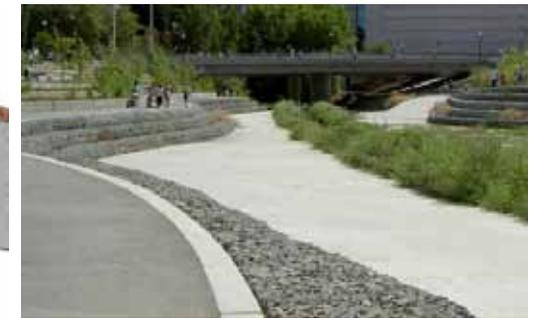
Example of permeable paving next to an asphalt pathway.
