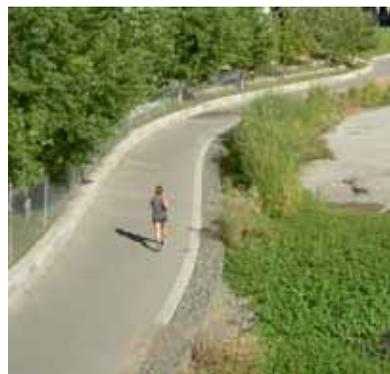
Asphalt trail with infiltration strip
