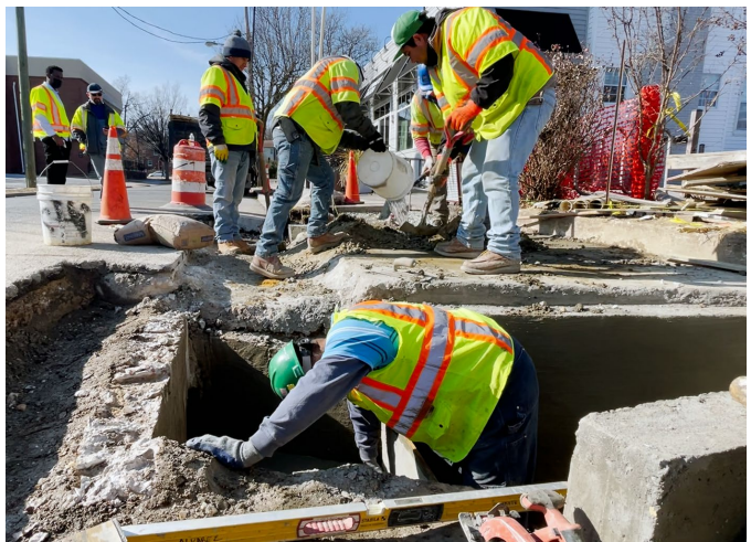
A crew pours concrete to form the catch basins for the new, wider inlets on Hume Avenue.
