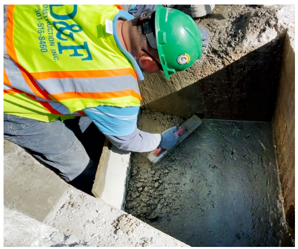
A crew pours concrete to form the catch basins for the new, wider inlets on Hume Avenue.
