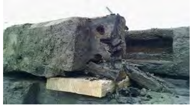
Above right: Detail of a mortise and tenon joint discovered while unloading the warehouse at the MAC Lab. Note the peg holes that run through this piece that would have secured the joint. Because of the dirt covering these beams, we had not previously seen this architectural feature. As the wood is cleaned at the MAC Lab, we expect to learn more about the architecture of this building.
