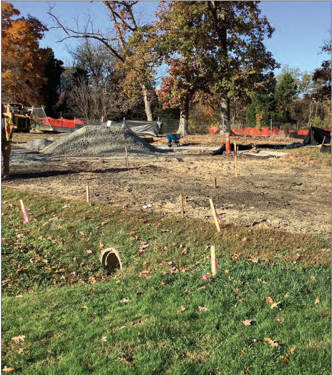
Figure 4. Culvert underneath Road, View North
