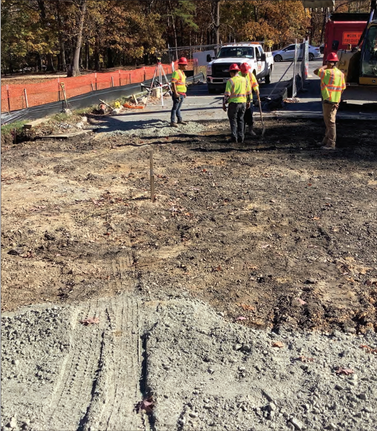
Figure 3. Road Base after Asphalt Removal, View East
