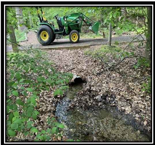
Park staff removed logs, leaves, and debris to clear storm drain. Dora Kelly Park
