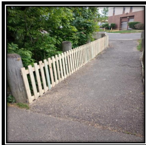
Holmes Run fence replace by staff Holmes Run Park
